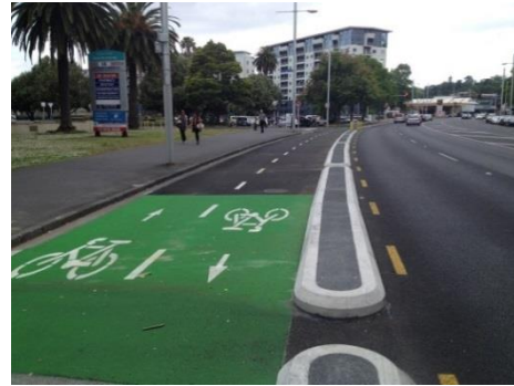
Figure 4: Protected cycle lane (bi-directional)
