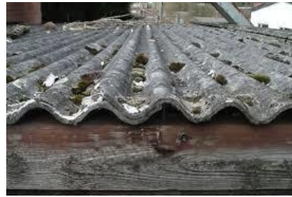
Figure 2: Asbestos roofing
