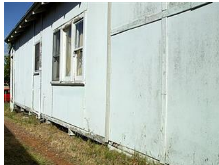
Figure 6: Asbestos cladding
