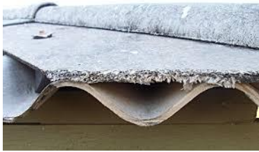
Figure 3: Asbestos roofing
